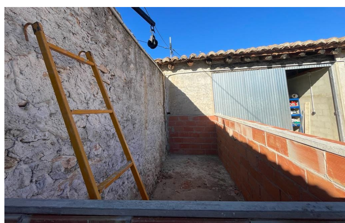
Fig. 2. Feedstock tank in construction phase
