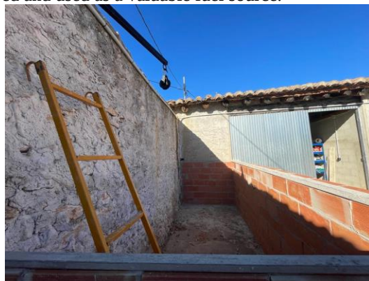
Fig.1. Feedstock tank in construction phase.
