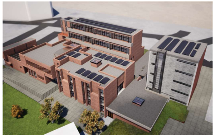
Fig.3. Aerial view of the PV deployment of 228 PV units of 385 Wp according to architectural criteria (authors).
