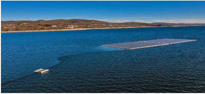
Fig. 2 . FSPV System in Dam Rabagão
