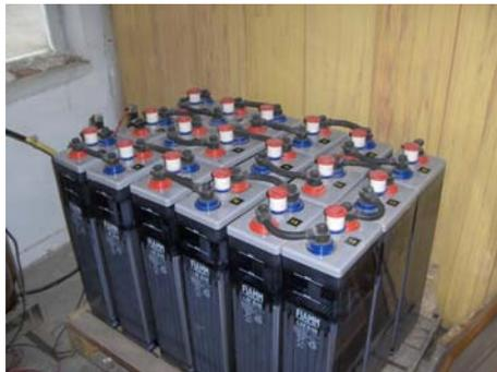
Figure 9-Batteries used as load
