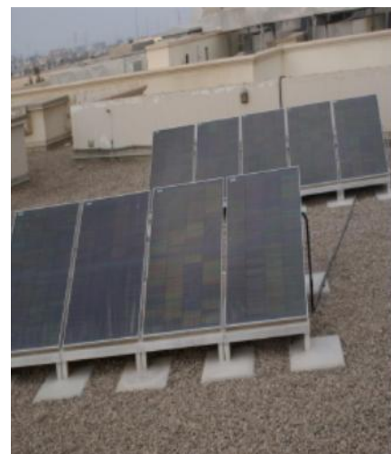
(a) (b) Figure 1: (a) A dusty day in the golf, (b) Roof-top panels affected by dust [12].
