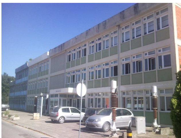
Fig.2. Main façade of the departmental building.
