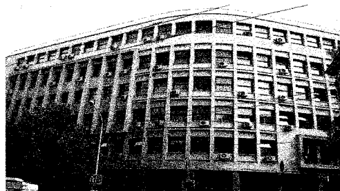
Fig. 1: An office building in Belgrade having many single phase split-type air conditioners installed
