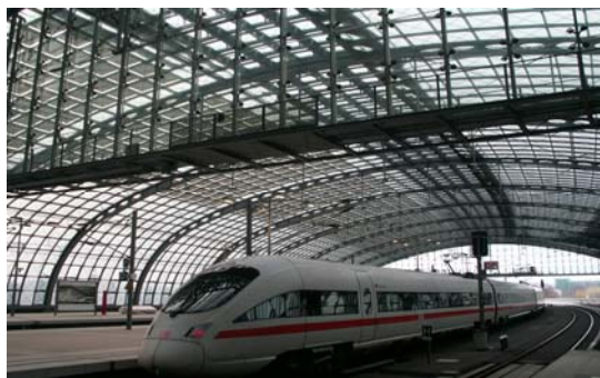
Fig 5. Lehrter Railway Station in Berlin - the PV modules [foto from author]
