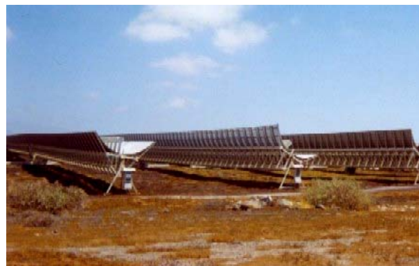
Fig. 6. .PV - installation with concentrators and one axis trackers in Instytutó Tecnológico Energie Renovable (ITER) on Tenerife [foto from author]
