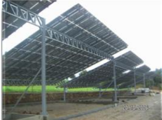
Fig. 11 Parking roof top (Ferreira do Zêzere, Portugal)
