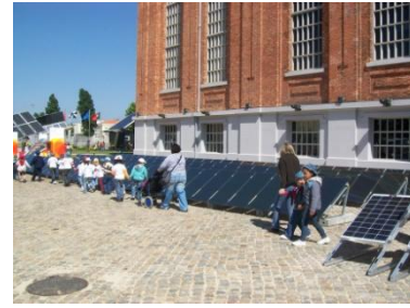
Fig. 12 View of the installation during the Solar Festival
