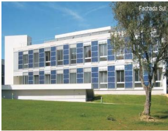
Fig. 10 Building second skin (INETI, Lisbon)
