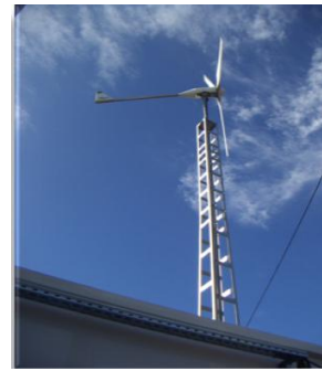
Fig 8. Wind turbine installation
