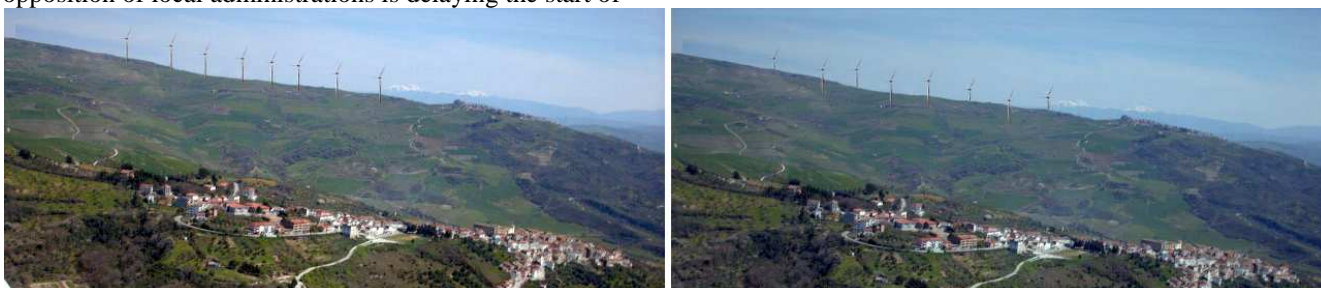
Fig.8. A different way to locate wind towers. The second image underline that a localization riding the ridges is better than a linear one on the top of the ridges.
