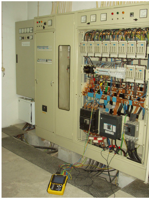
Fig. 4. Collecting data with power analyser.
