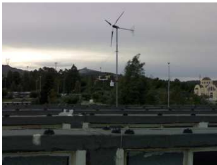
Fig. 1. W/G on the roof of L.E.M.E.C
