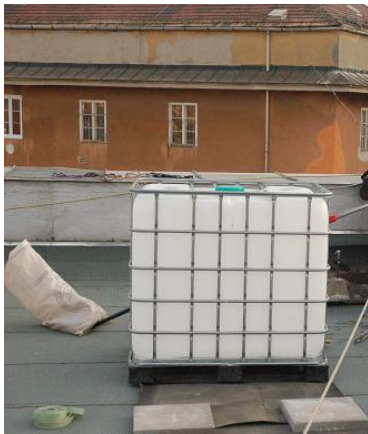
Figure 7.: The upper reservoir
