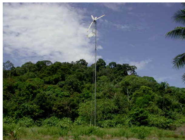
Fig. 3: Small wind turbine on high pole damaged by lightning.
