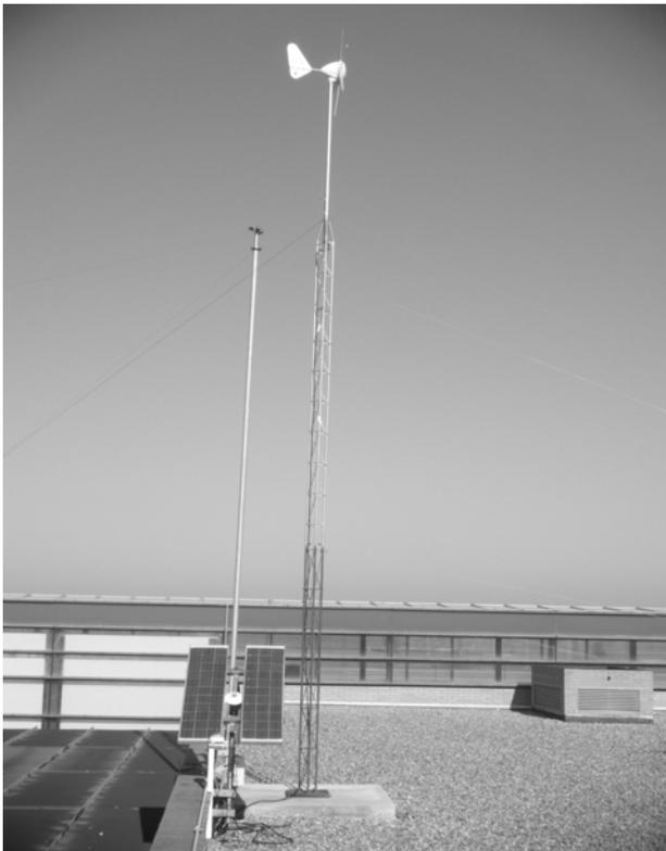
Figure 3. Wind – solar generator
