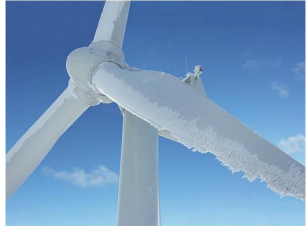
Fig. 7. Ice on a wind turbine blade [10]
