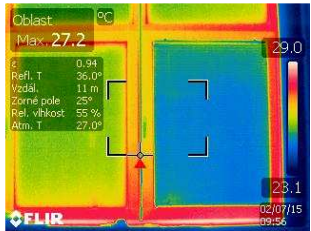
Fig. 5. Sample thermogram (5 th floor, room EL511 - S).
