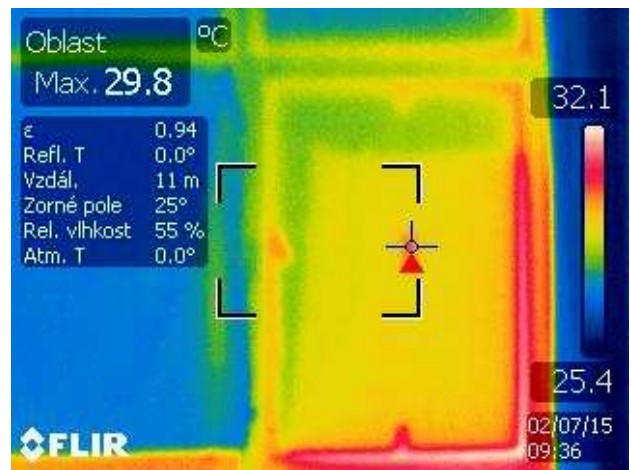
Fig. 4. Sample thermogram (3 rd floor, room EL311 - S).
