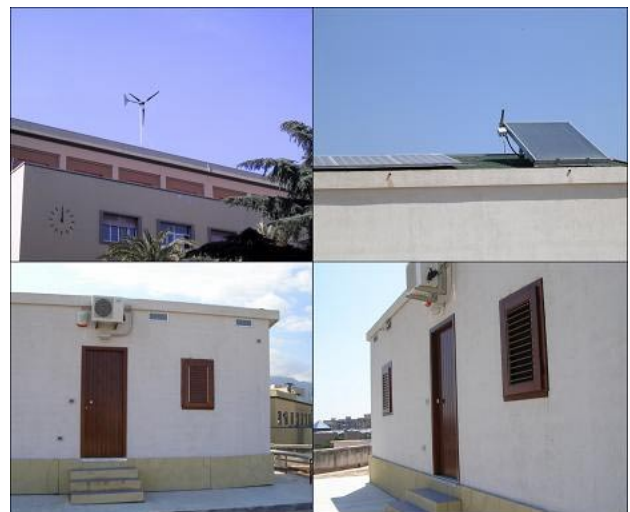
Fig. 1. The mobile house, the wind microturbine and the PV field.
