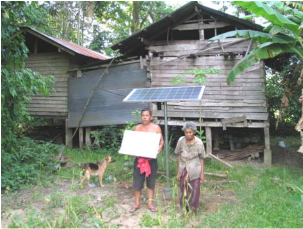
Fig. 5 Typical SHS implementation in Thailand with fixed mounting of PV modules (Photograph: Courtesy Solartron Co., Ltd.)
