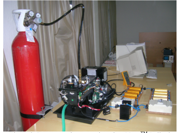
Figure 3. Power supply system based on Nexa™ Ballard module in our laboratory.
