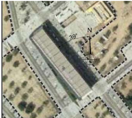
Fig. 2. Orientation of Building 17.
