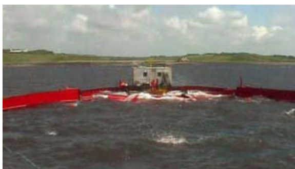
Fig. 10 Wave Dragon System Installation Nearshore
