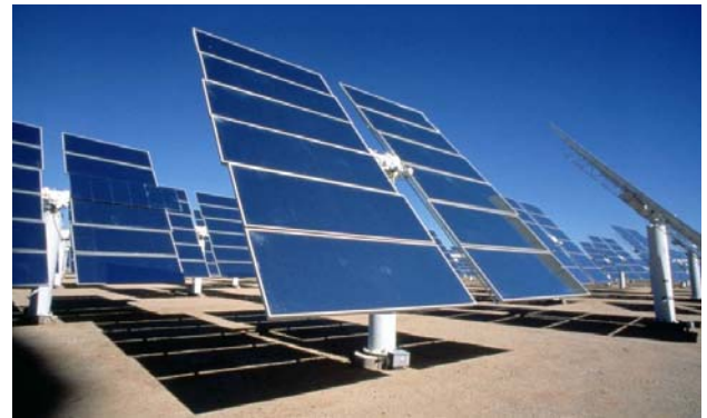
Fig. 21. Photovoltaic panels. (Courtesy of [13])
