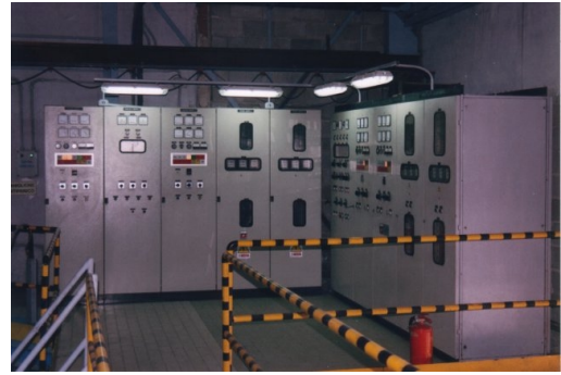
Fig. 3. Medium-voltage switchboards
