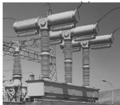
Figure 9. Double break 168kV/31,5kAVCB [13]
