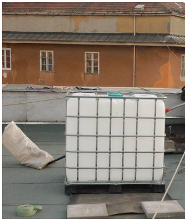
Figure 7.: The upper reservoir
