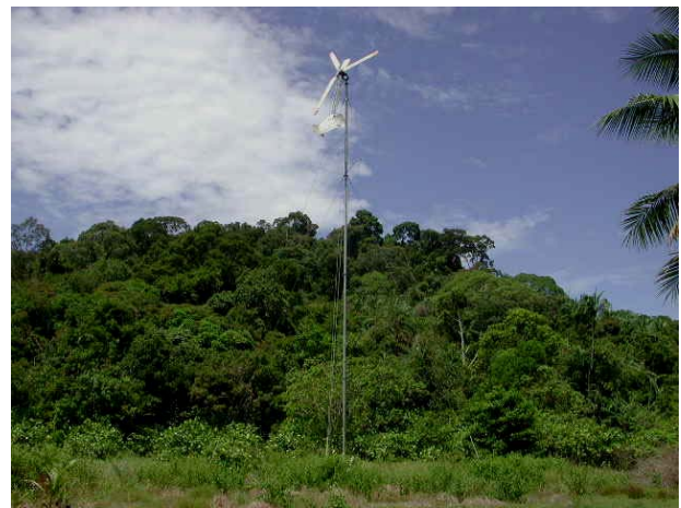
Fig. 3: Small wind turbine on high pole damaged by lightning.
