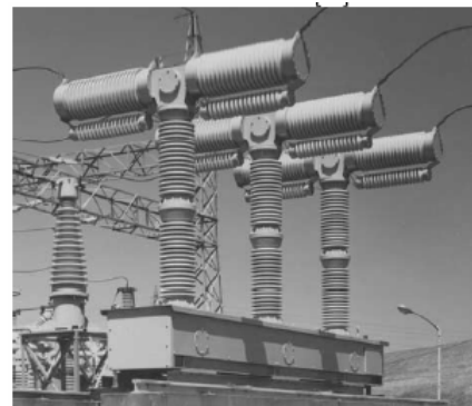
Figure 9. Double break 168kV/31,5kAVCB [13]
