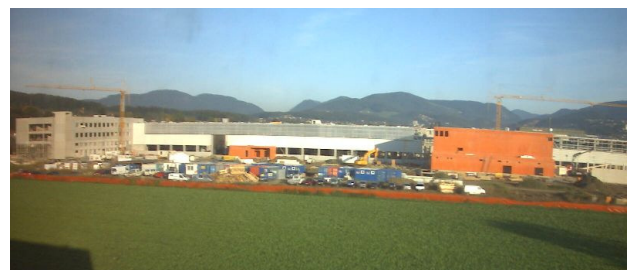
Fig. 1. View of the new manufacturing plant for electrical machines, September 2008.
